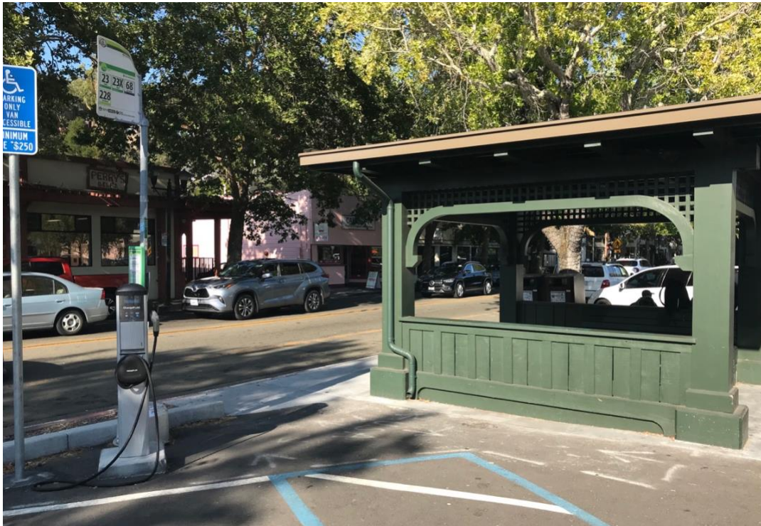
Downtown Fairfax ADA electric vehicle charging site and transit stop
