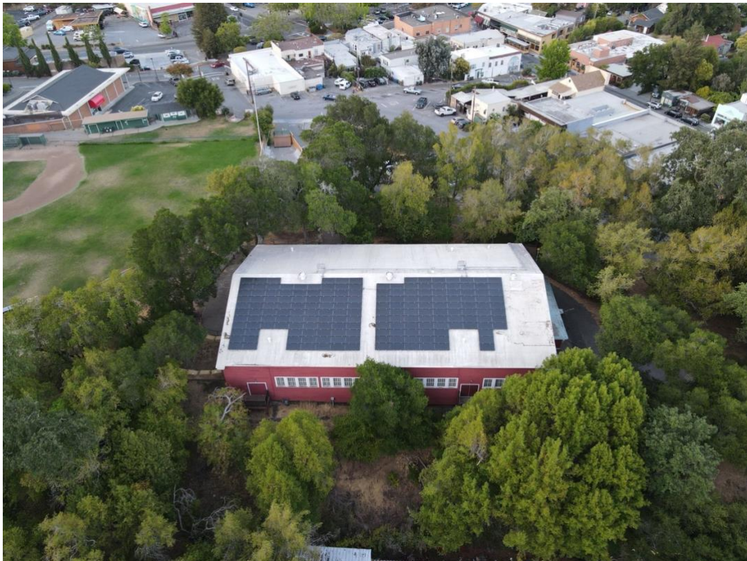
Fairfax Pavilion solar array ( photo by Rod Milstead )
